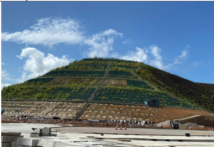
Hydro-seeding was applied on the slope to minimize muddy runoff.
