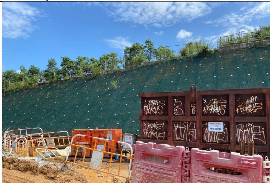
Hydro-seeding was applied on the slope to minimize muddy runoff.
