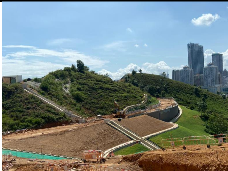
The completed slope surfaces were compacted and hydroseeded.
