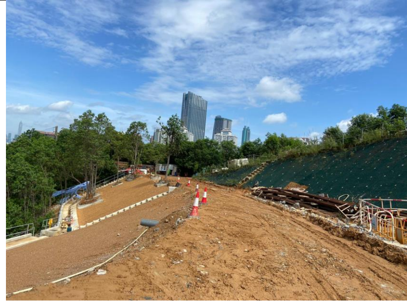
Runoff would be collected by the built surface u-channel and diverted to the soakaway trench.
