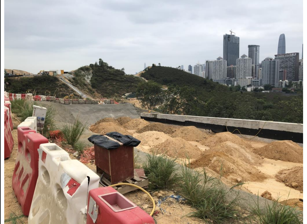
Exposed slopes surface was paved by cement mortar to minimize muddy runoff.
