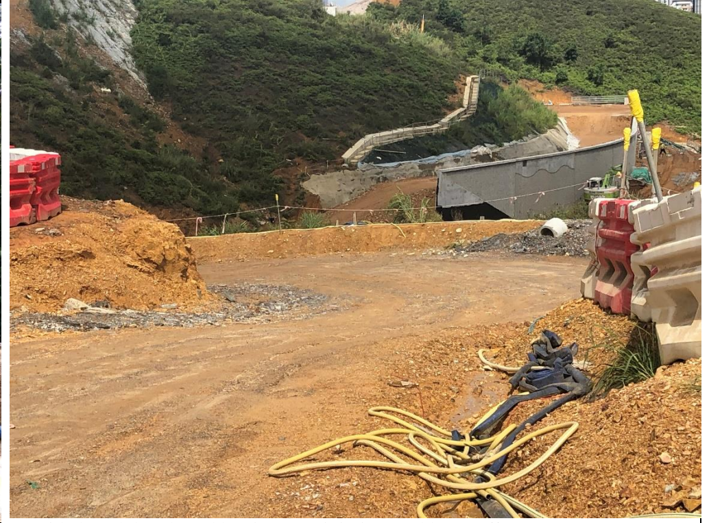
Provided earth bunds and barriers to minimize muddy runoff.
