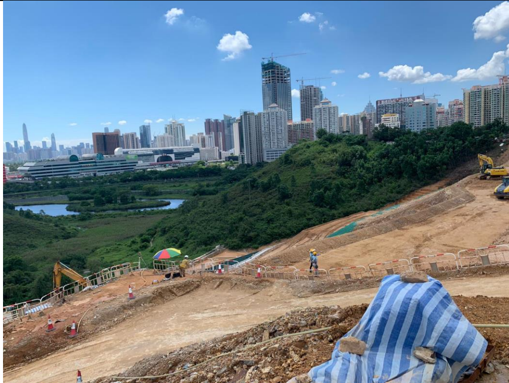
Provided efficient silt removal facilities to prevent leakage of muddy runoff from site area. Removal of silt was conducted by the Contractor regularly.
