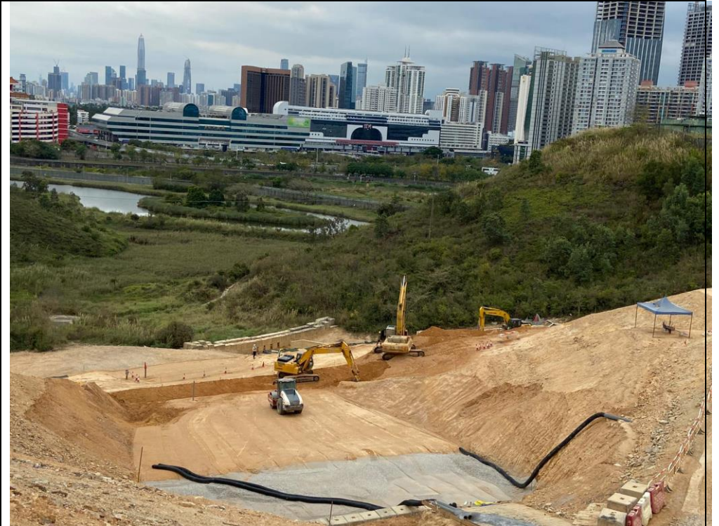
Temporary drainage was provided to prevent runoff going through site surface.
