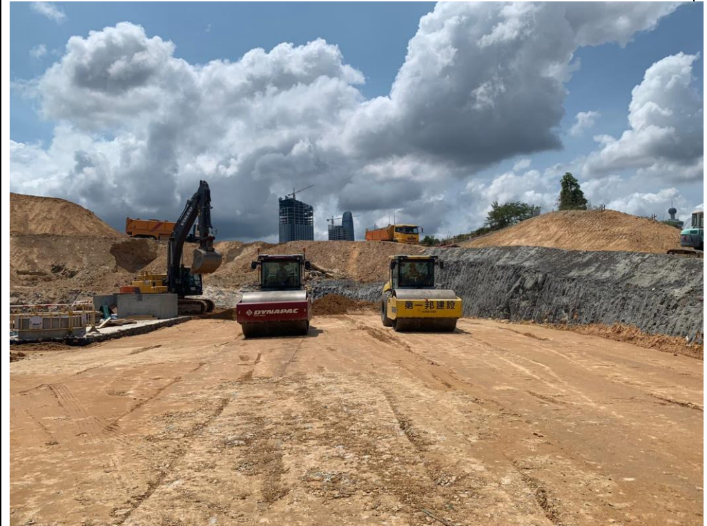
Exposed slopes surface were covered by cement mortar
