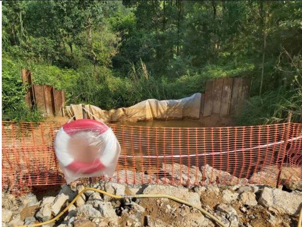
Sump pit and geo-textile were installed to prevent leakage of muddy runoff at Area Part A1.
