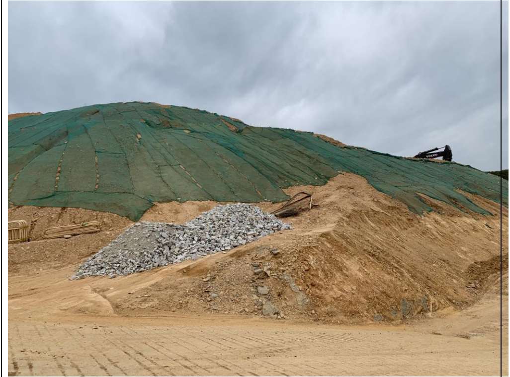
Exposed slopes surface were compacted and covered.
