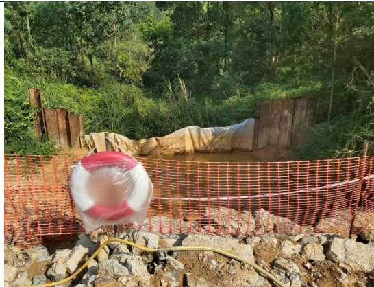
Sump pit and geo-textile were installed to prevent leakage of muddy runoff at Area Part A1.
