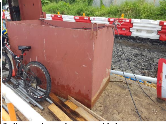
Sedimentation tank was provided to treat any wastewater at TTA2.
