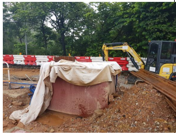
Sedimentation tank was provided to treat any wastewater at TTA1.
