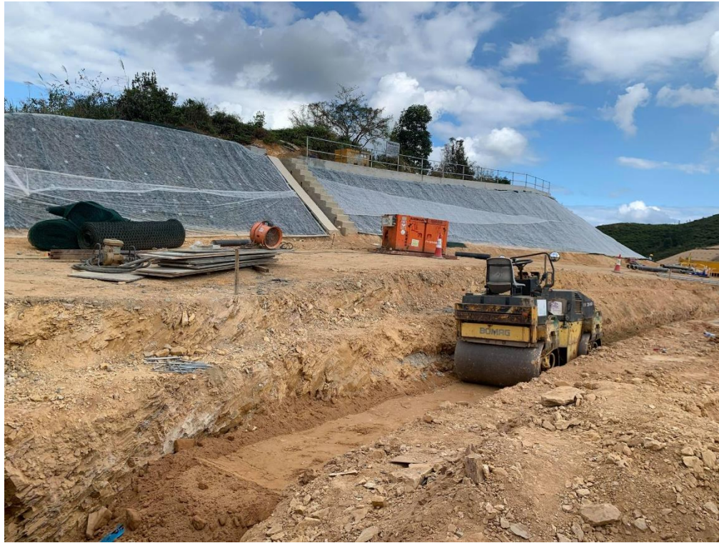
Hydro-seeding was applied on the slope to minimize muddy runoff.
