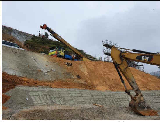
Exposed slopes surface was paved by cement mortar to minimize muddy runoff.
