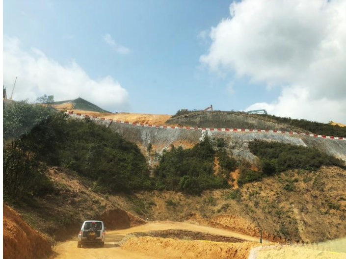
Exposed slopes surface was paved by cement mortar and provided earth bunds along the access road to minimize muddy runoff.
