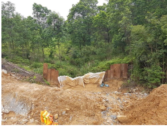
Sump pit and geo-textile were installed to prevent leakage of muddy runoff.
