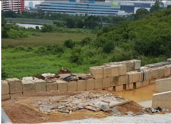
Provided efficient silt removal facilities to prevent leakage of muddy runoff from site area.
