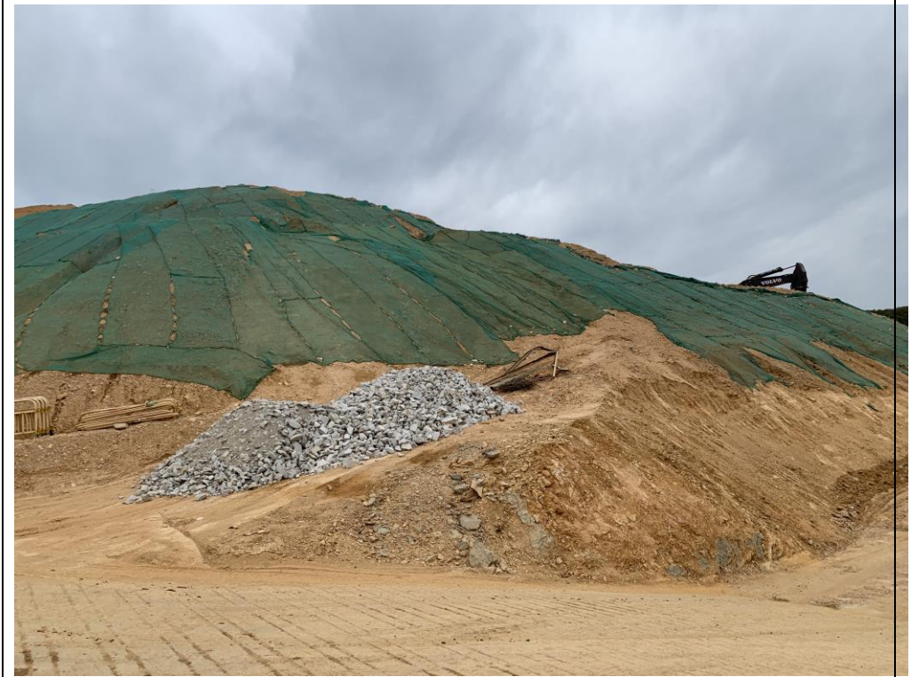
Exposed slopes surface were compacted and covered.
