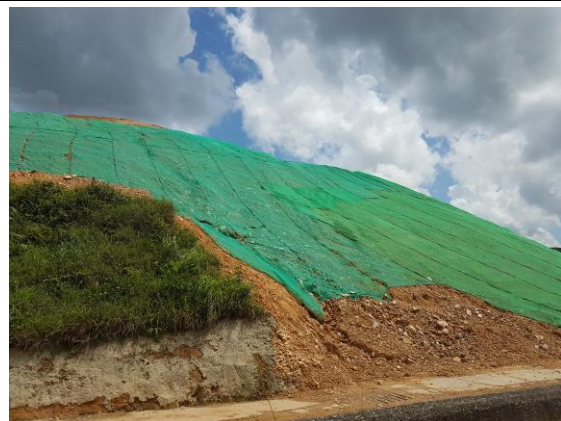
Exposed slopes surface were compacted and covered with tarpaulin sheet or similar means.
