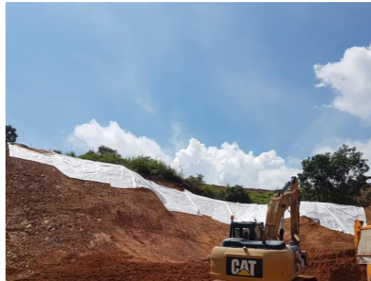
Exposed slopes surface was covered with tarpaulin sheet or similar means.
