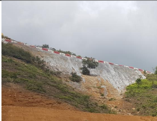
Exposed slopes surface was paved by cement mortar and provided earth bunds along the access road to minimize muddy runoff.
