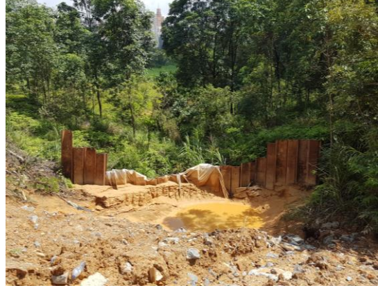
Sump pit and geo-textile were installed to prevent leakage of muddy runoff.
