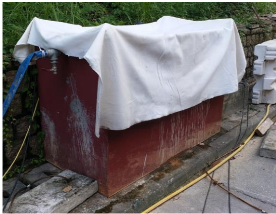
Sedimentation tank was provided to treat any wastewater at TTA2.
