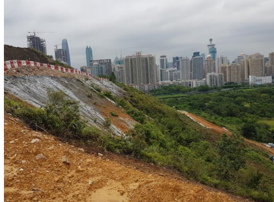
Exposed slopes surface was paved by cement mortar.
