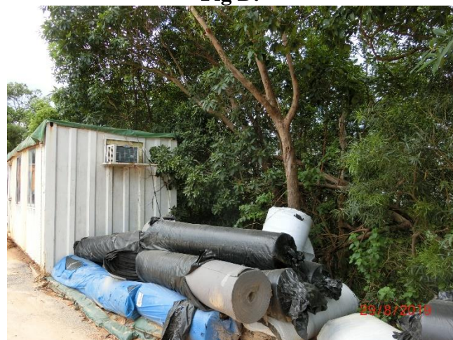
Tree protection zone is missing
