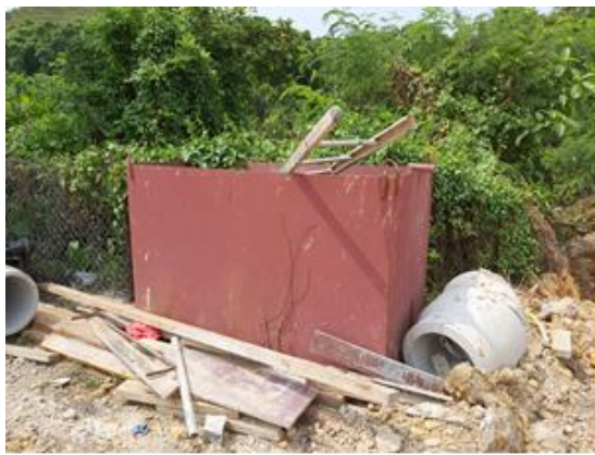
Sedimentation tank was provided to treat any wastewater at TTA1.
