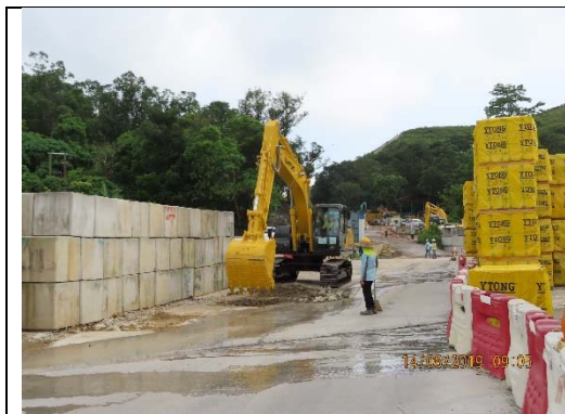
Pit excavation by Excavator
