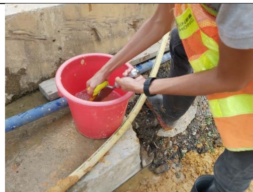
Cleaning of equipment with phosphate-free detergent (Decon® 90)
